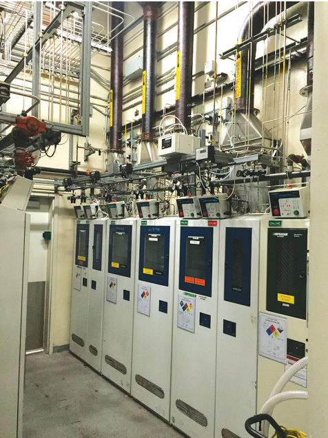
Figure 3. Toxic Gas Cabinets at Analog Devices' Wafer Fab are Closely Monitored to Ensure Uptime
