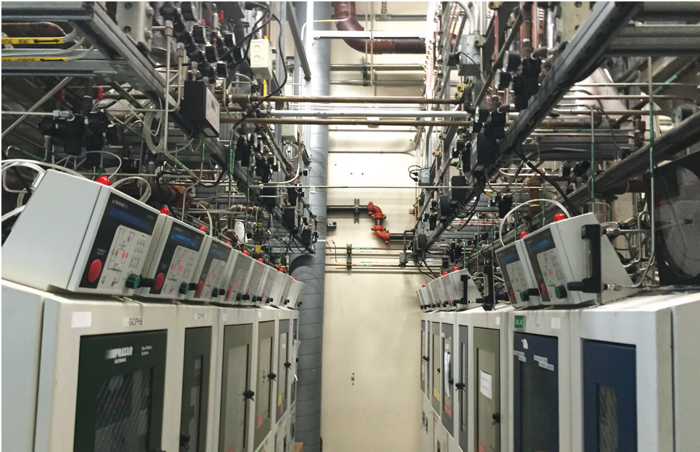
Figure 4. Dense Metal and Concrete—Wireless Nodes Must Perform Reliably Even When Located Among Metal Equipment and Gas Distribution Pipes
