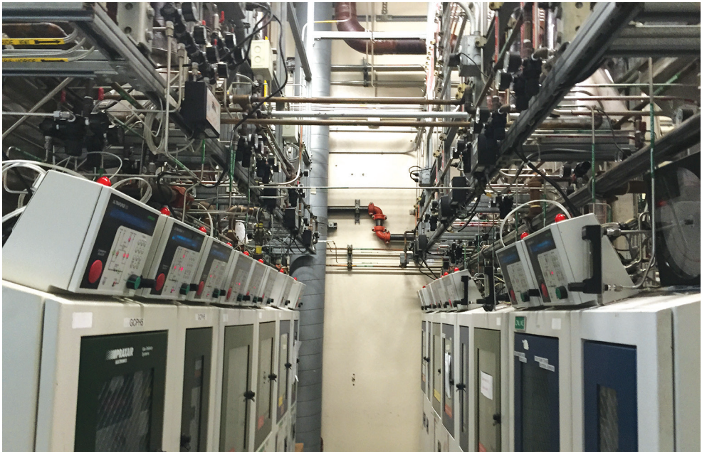
Figure 1. Dense Metal and Concrete—Wireless Nodes Must Perform Reliably Even When Located Among Metal Equipment and Gas Distribution Pipes
