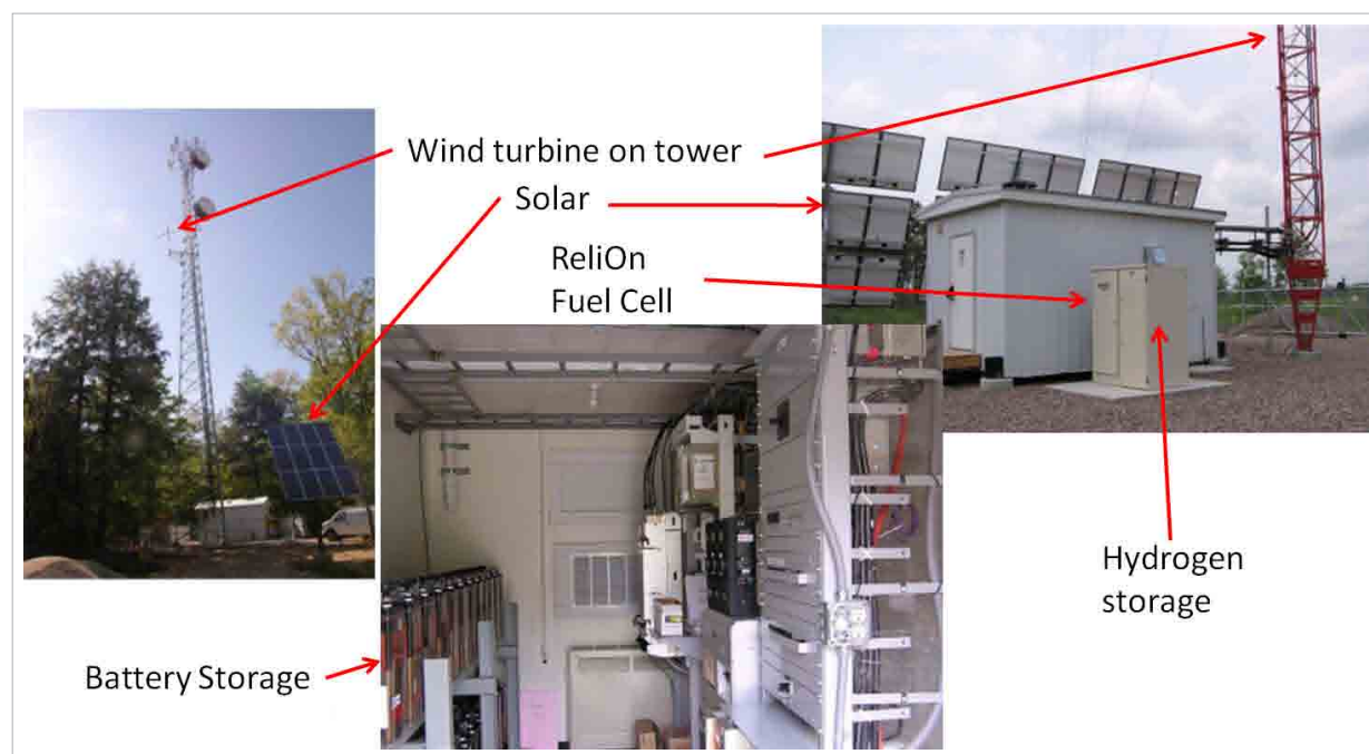
Figure 3: Switching from lead-acid to Li-ion batteries makes room for more telecom equipment in an off-grid hybrid site operating from batteries, wind, solar, and fuel-cell technology. (image courtesy A123 Systems)
